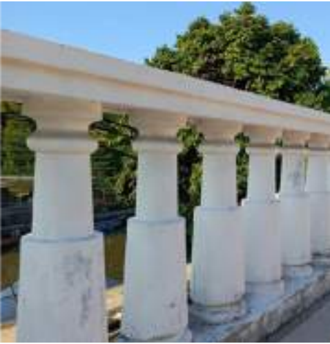
Gambar: Railling/Balustrade Beton Area Teras Belakang
